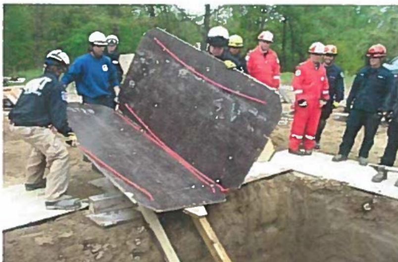
Panel Squad 2 on Wall 2 setting the Corner Panel onto rails to slide into the trench and place on Corner Wall# 1
