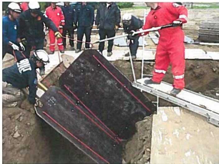
Panel Squad # 1 receiving the Corner Panel
