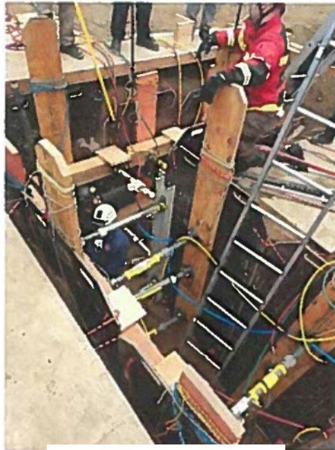
Secondary Shoring in Place
