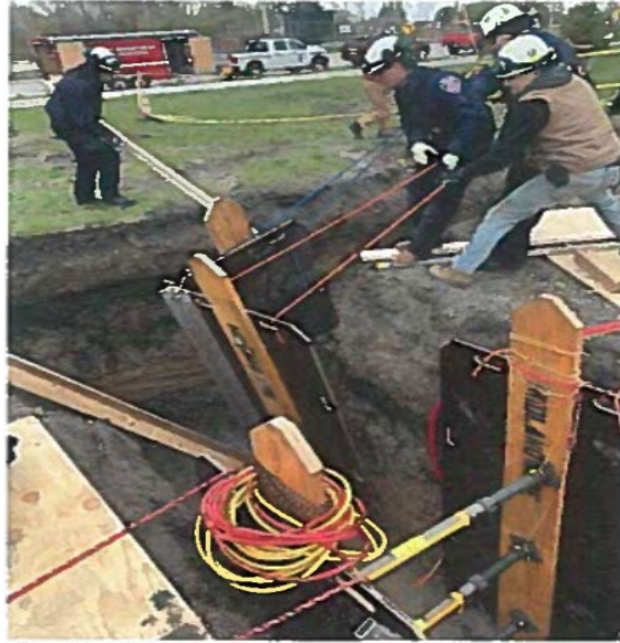
Panel Squad # 1 positioning the Corner Panel
